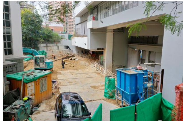
Ariel Photos in February 2022 - All piles were completed. Ground is temporarily backfilled to prepare for statutory loading test to ensure the integrity of piles.
