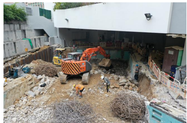
Ariel Photos in June 2021 - Swimming pool is being demolished.
