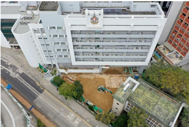
Ariel Photos in February 2022 - All piles were completed. Ground is temporarily backfilled to prepare for statutory loading test to ensure the integrity of piles.
